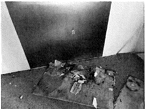
Damaged Tiles
